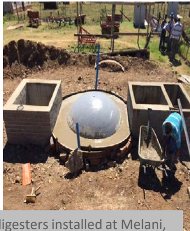
10m 3 Balloon-type digesters installed at Krwakrwa and Melani villages in the Eastern Cape
